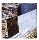
Program to design and check reinforced cantilever walls for soil retention. An automatic geometric pre-design is carried out as well as the section reinforcement and geometric and reinforcement design of the wall foundation.
